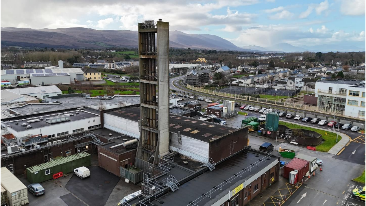
Figure 1 - Exhaust Flue Chimney
