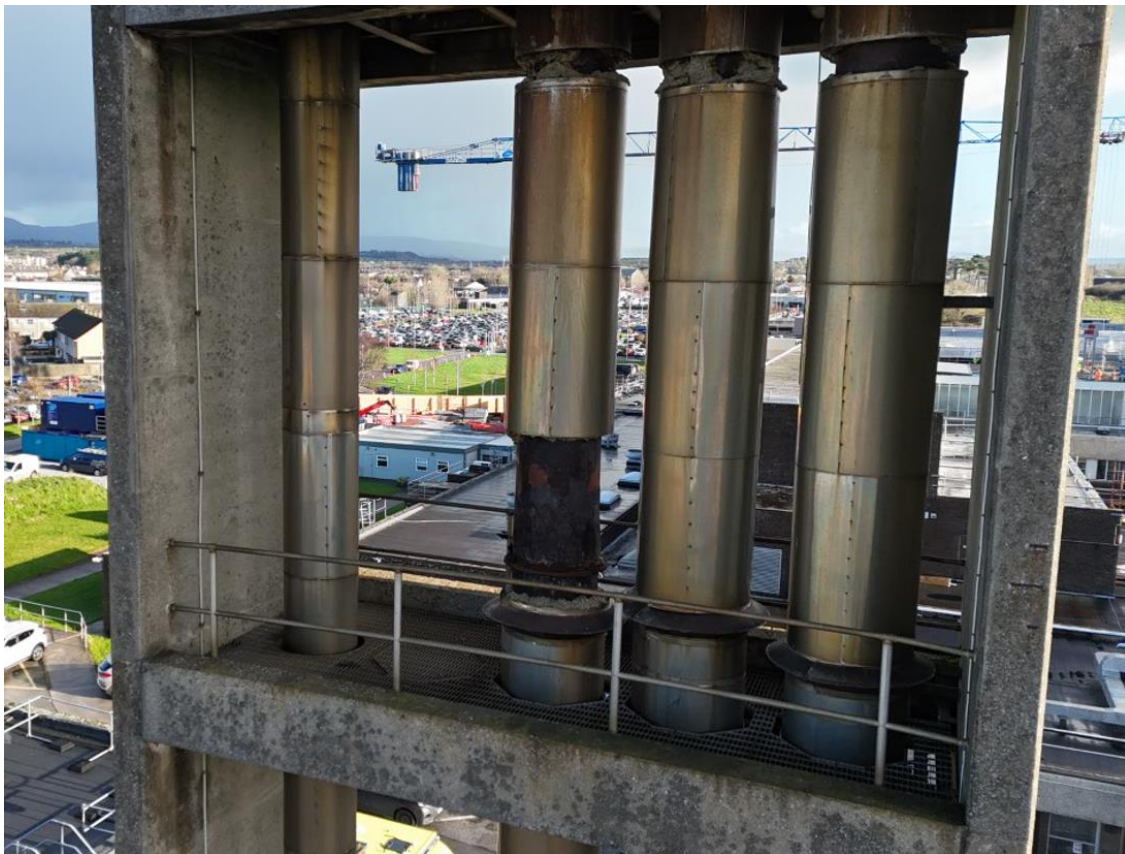
Figure 5 - Flue stacks supported within chimney. Extensive rust visible on central flue where cladding is missing.
