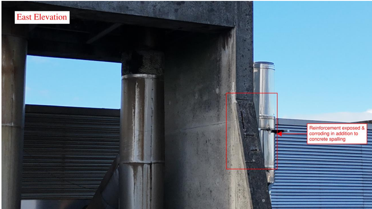
Figure A. 15 - Concrete defects on east elevation
