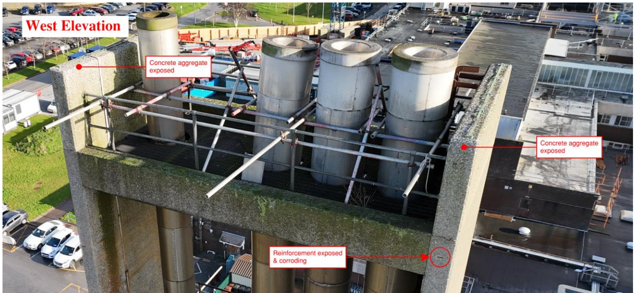
Figure A. 9 - - Concrete defects on west elevation
