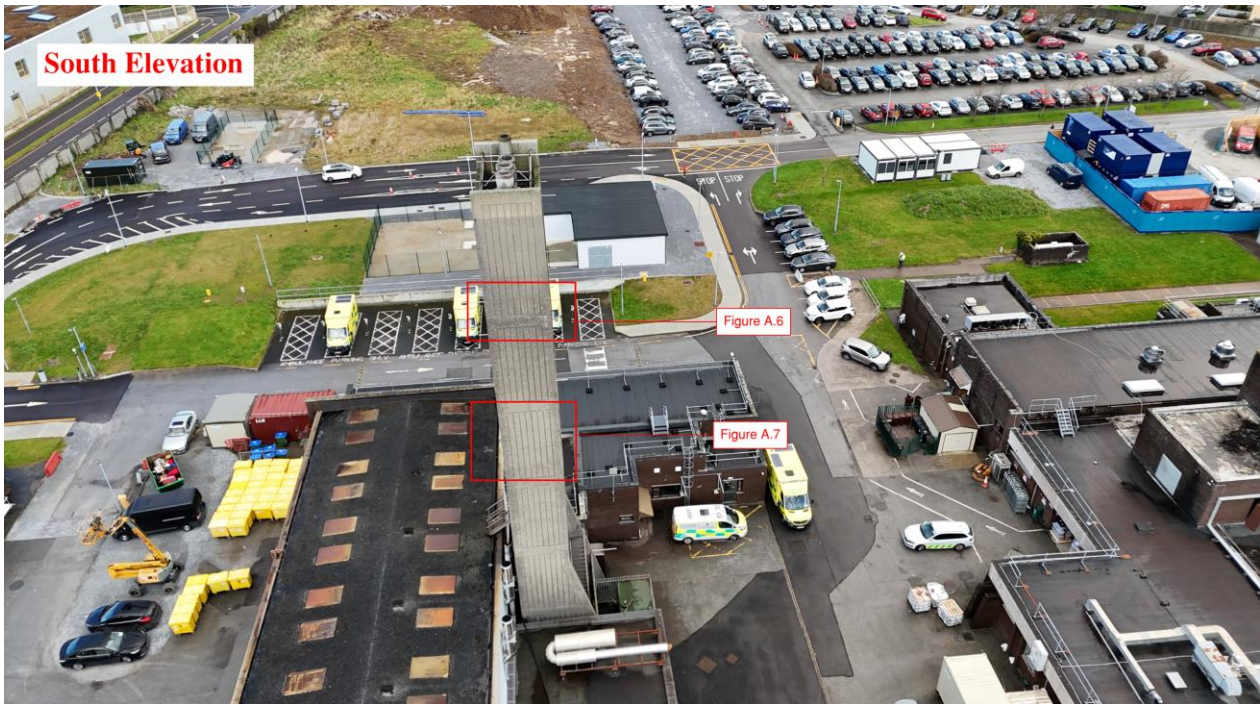
Figure A. 5 - Chimney south elevation
