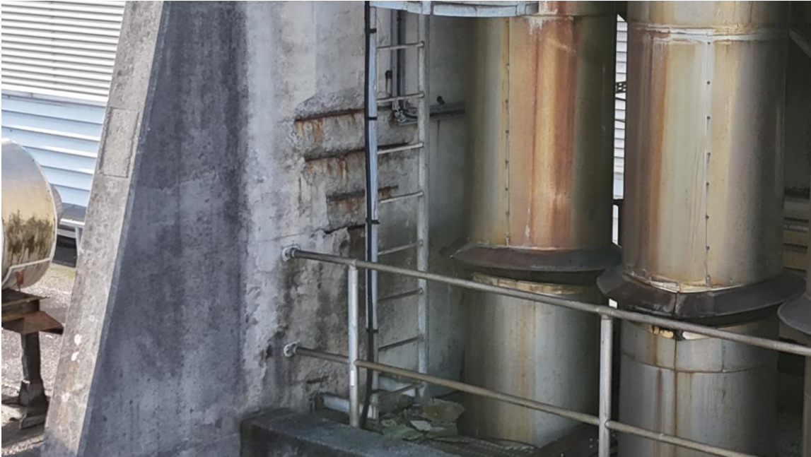
Figure 2 - Spalling concrete and exposed, corroding reinforcement at first platform level
