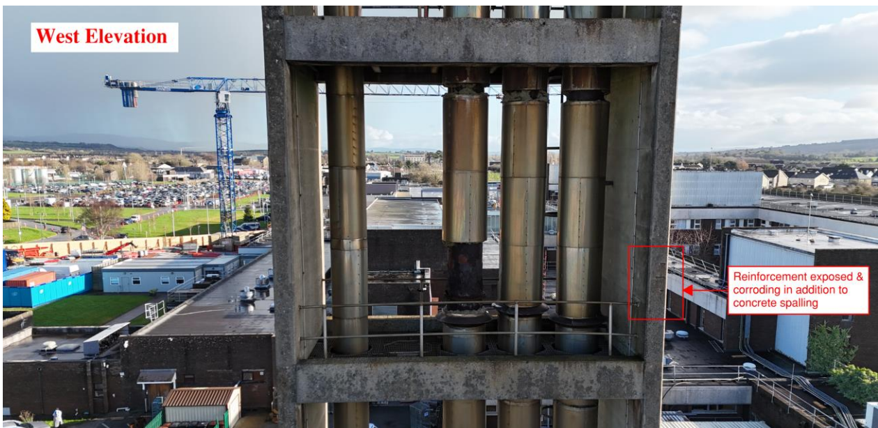
Figure A. 12 - Concrete defects on west elevation
