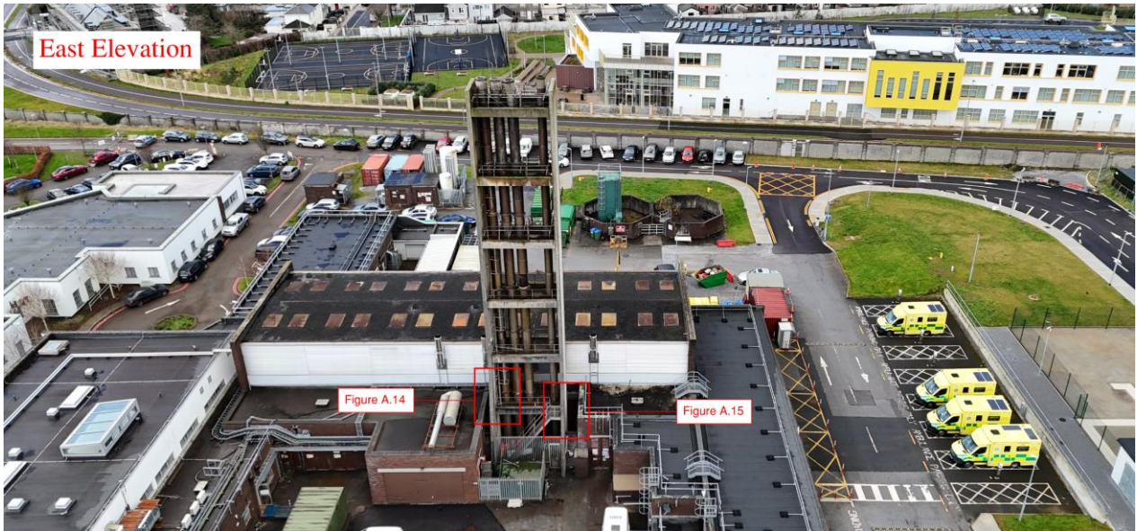
Figure A. 13 - East chimney elevation
